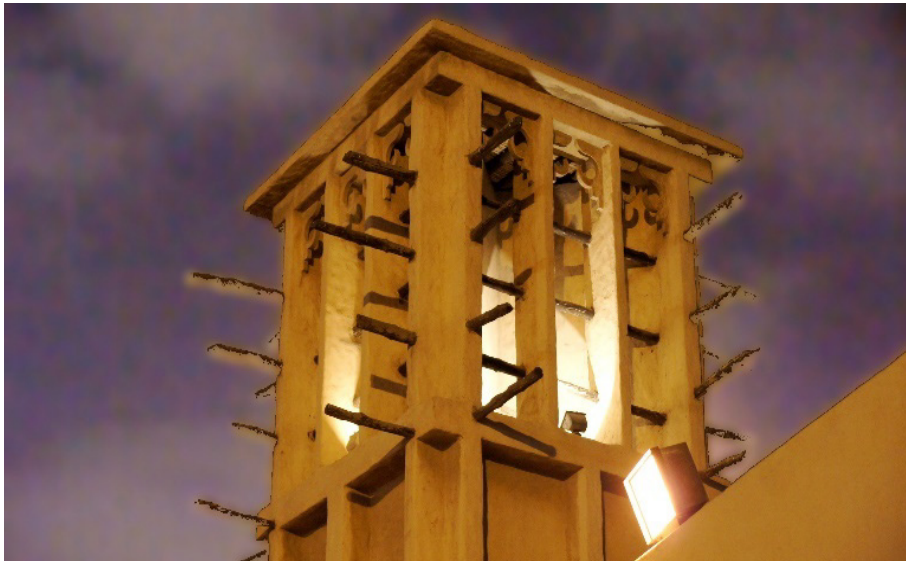
Figure 13. Emirati windcatcher (picture taken by the author, October 2009, Dubai, UAE).
